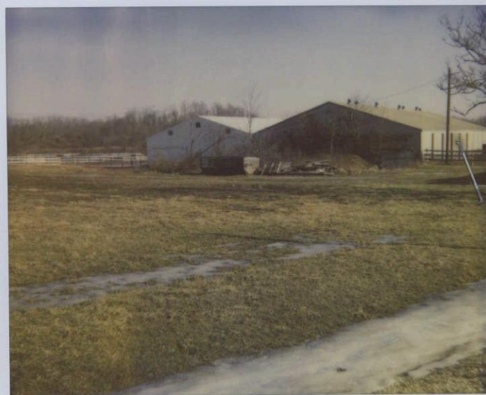
WEST SIDE PARKING AREA
